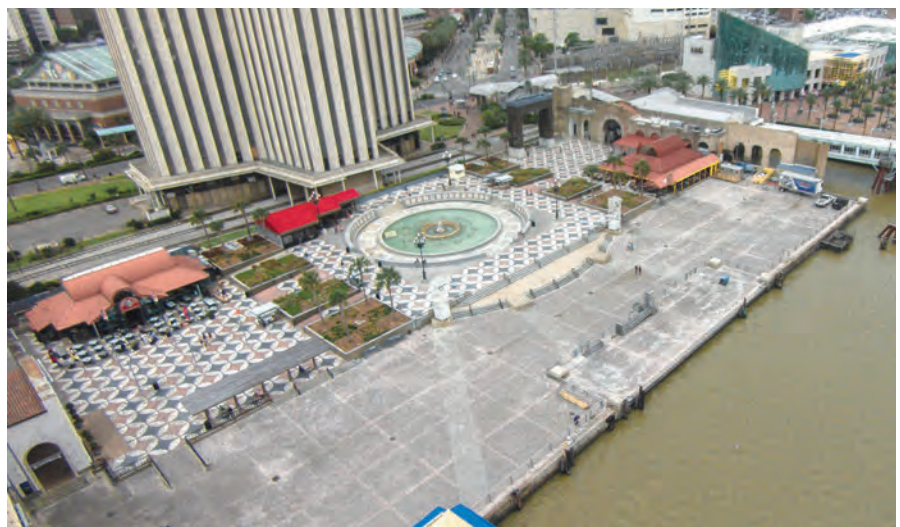
Lack of shade throughout Spanish Plaza and the Canal Street Wharf
