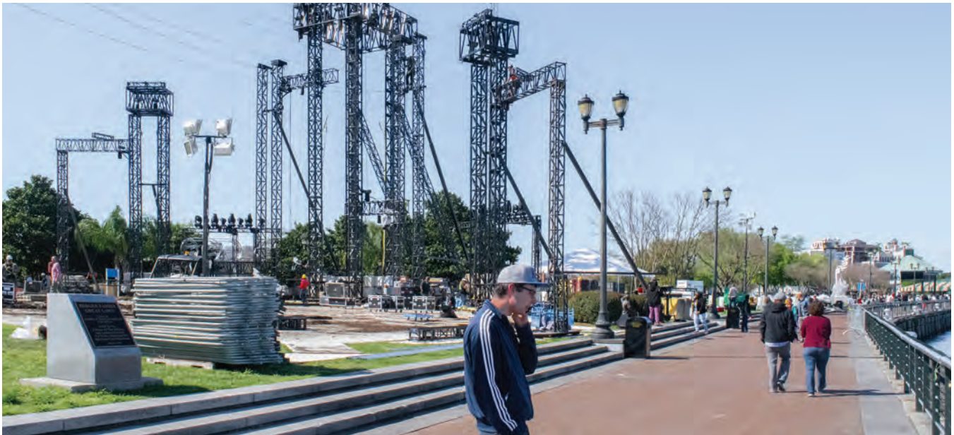
Spaces along the riverfront being utilized for festivals events ensuring the need for proper programming
