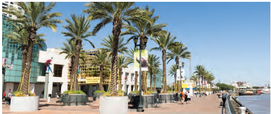
View looking downriver featuring grid of palm trees and planters set back from the river to form the Promenade
