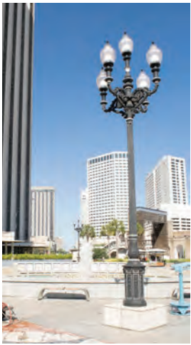
Large light poles
