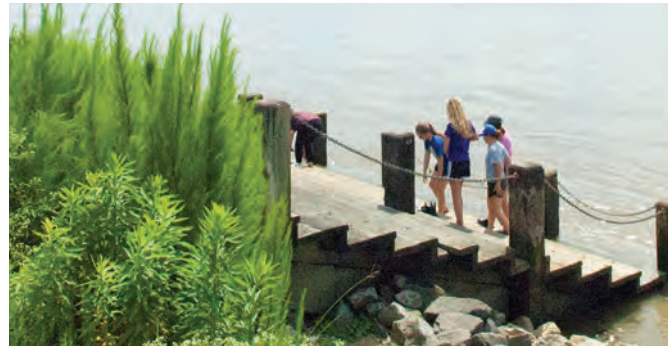
Wooden steps provide safe access to the river
