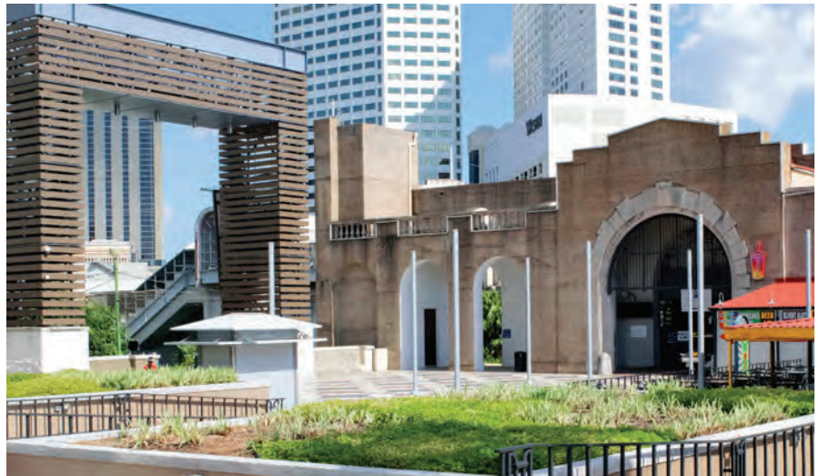
Canal Street access into Spanish Plaza and Ferry Terminal arcade entrances side by side
