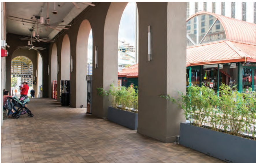
Planters, vending machines, and the Time Out Restaurant impede circulation
